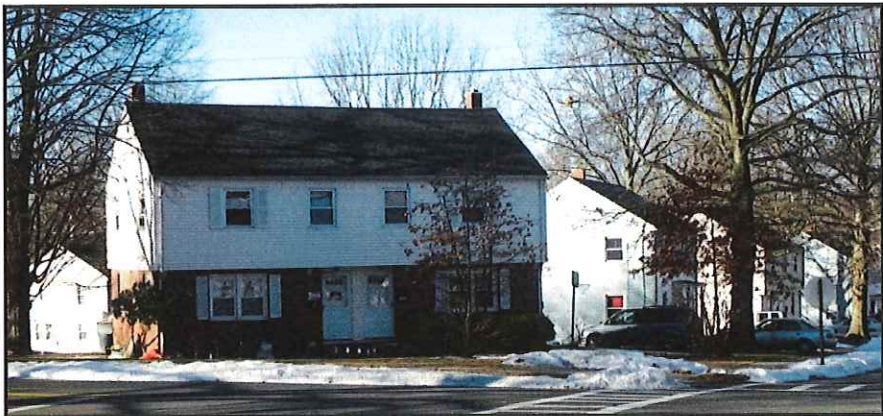
Green Valley Drive by Pearl Street
