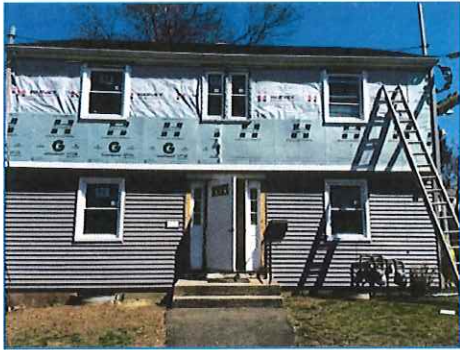
Siding & Window Upgrades
