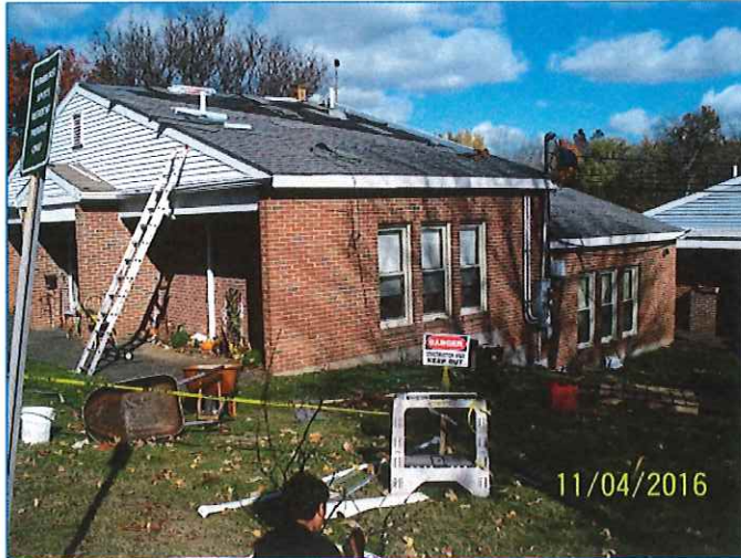
Roofing at Windsor Court
