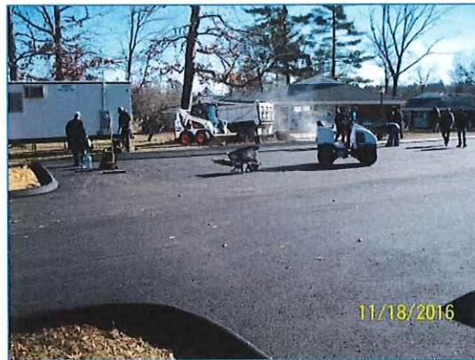
Paving at Woodside Park
