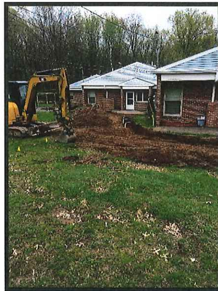
Alarm System Trenching
