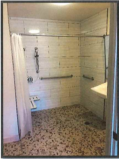
Accessible Shower Upgrade
