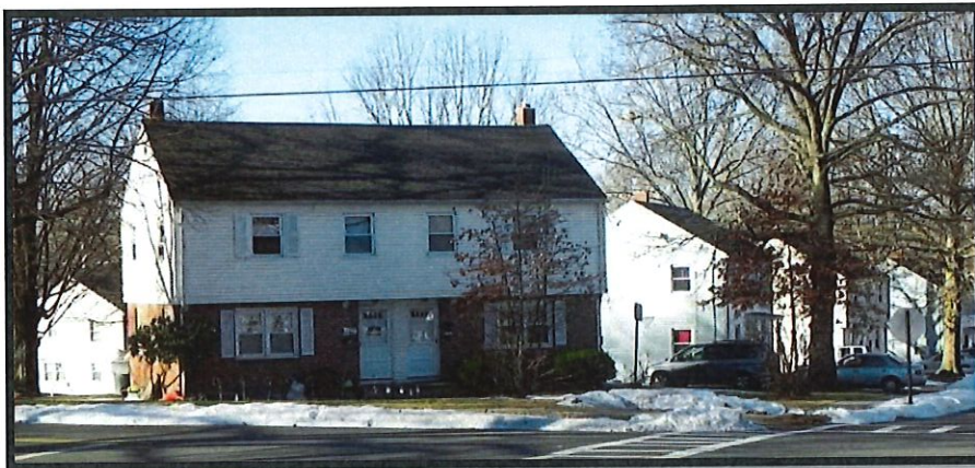
Green Valley Drive by Pearl Street
