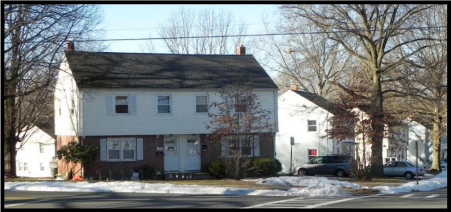
Green Valley Drive by Pearl Street
