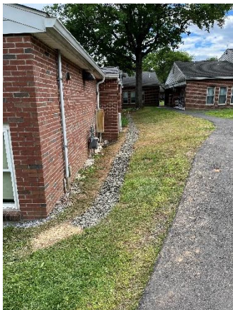
Windsor Court French Drain Installation
